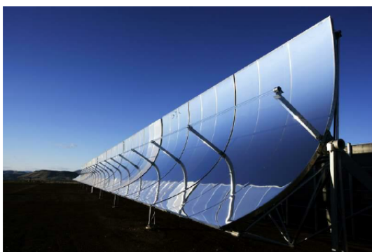
(e) Parabolic trough solar collector [18].
