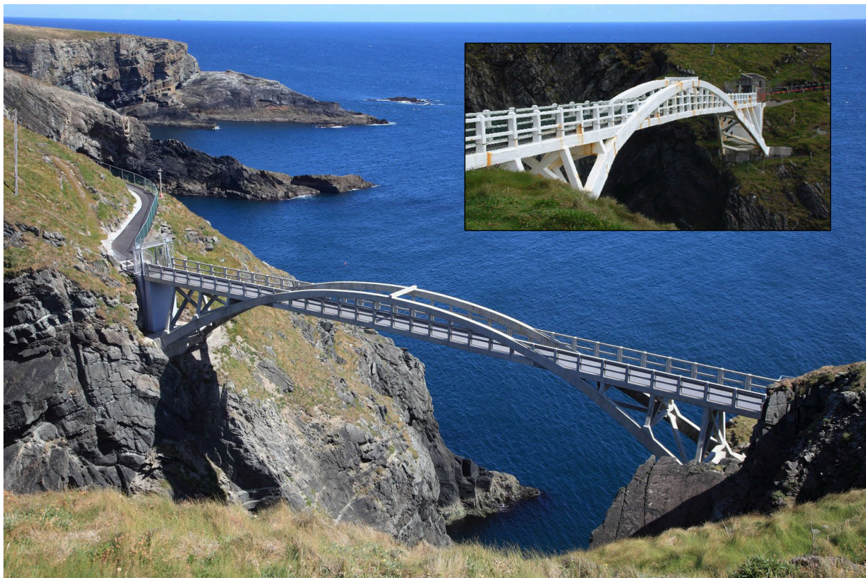
Figure 9.16: The newly constructed replica of the Mizen head bridge, county Cork Ireland and an insert of the original bridge constructed in 1909, (main photo from http://apresidentsblogbyppjrudden.blogspot.fr and insert by ©C.W. Glynn, licensed for reuse under the Creative Commons Licence).
