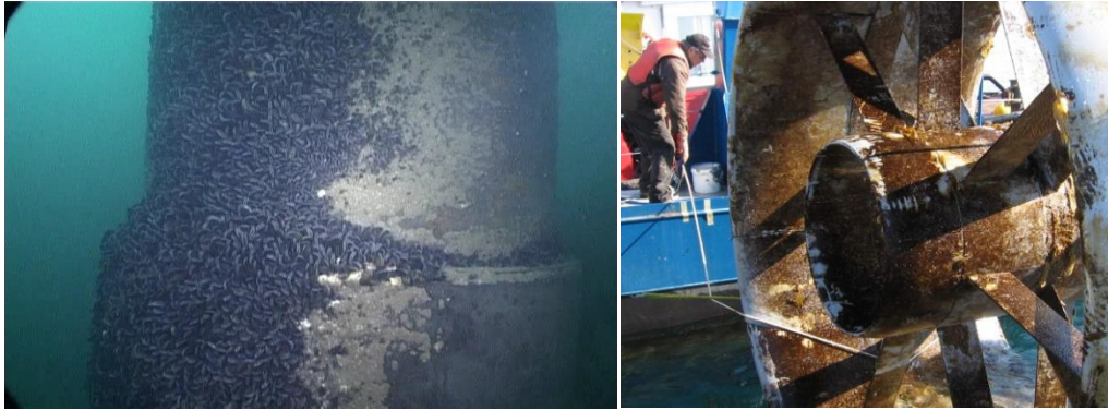
Fig.I.16 Biofouling & Erosion for MCECS [24]
