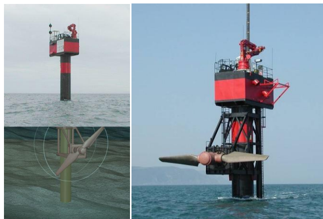
Fig.I.6 Seaflow, world's first MCECS pilot project at a commercial scale [5]
