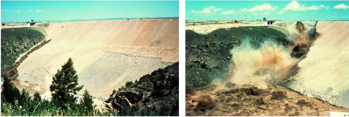
**Figure 1 Failure of Teton dam**
