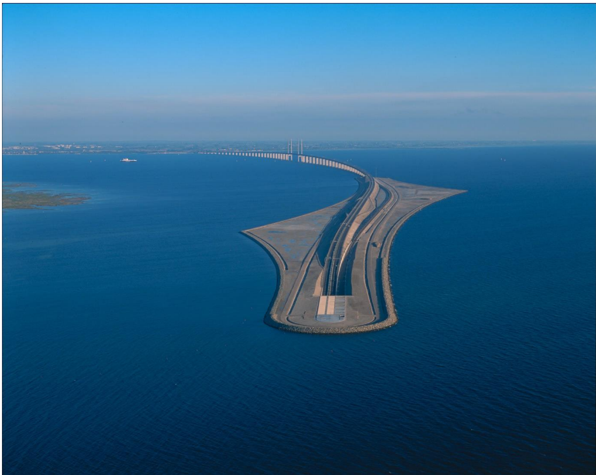
Figure 1.1 The Øresund Bridge between Denmark and Sweden dips into a tunnel through an artificial island called Peberholm
